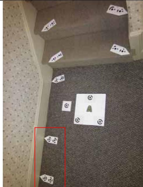
**4- For the free standing hand rail side of the stairs, position markers to indicate the plumb position of the railing. (use of plumb bob is shown)**
